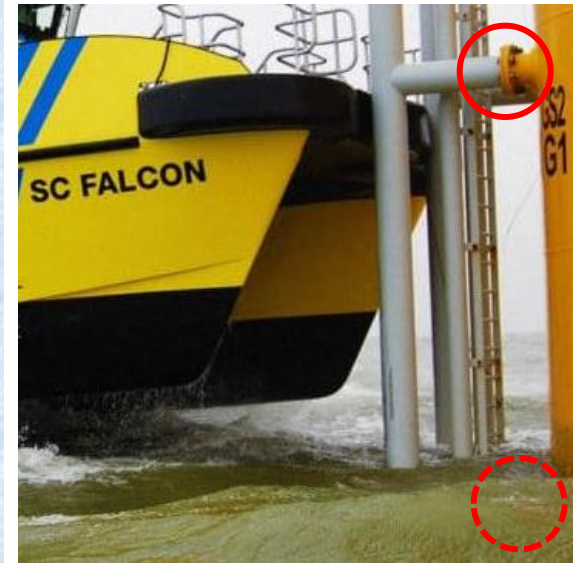
Flanschverbindung an Offshore Boatlanding
